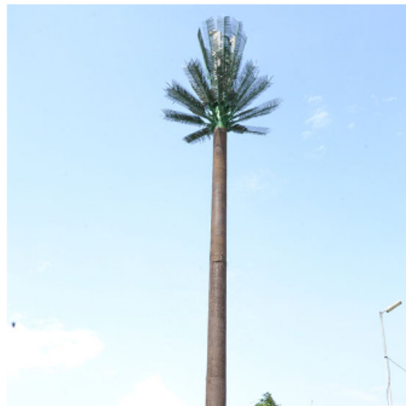
Telecommunication Palm Tree Steel Monopole Tower
