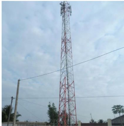
3 legs angular telecom steel tower
