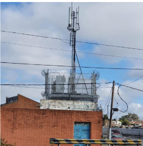
Hot dip galvanized Rooftop tower
